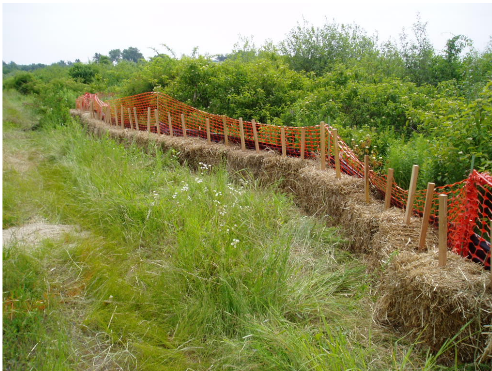
Photograph 2 – Silt Fence with Straw Bales and Construction Fence
