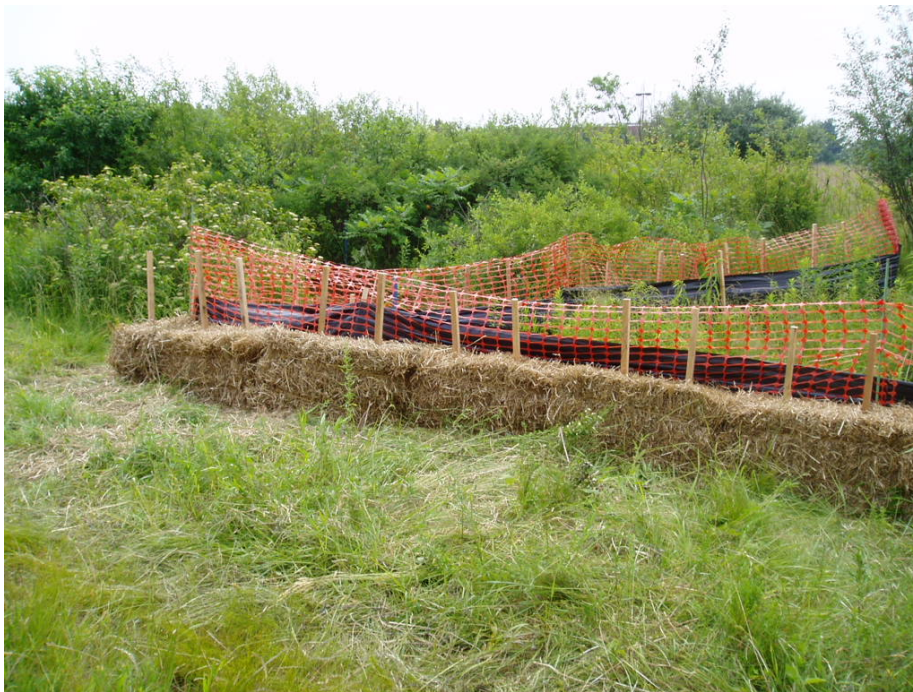
Photograph 3 – Silt Fence with Straw Bales and Construction Fence
