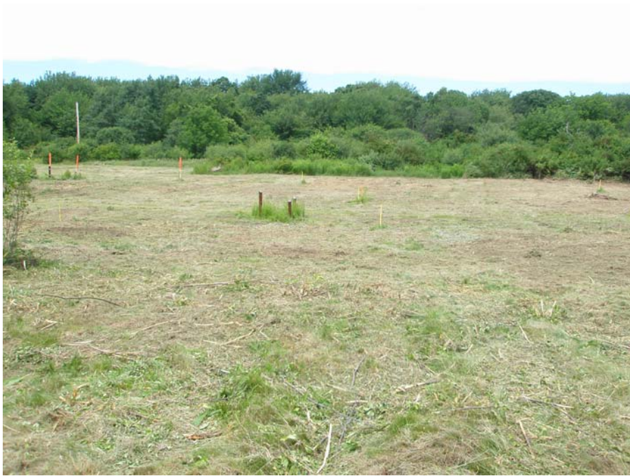
Photograph 5 – Cleared Excavation Footprint Area
